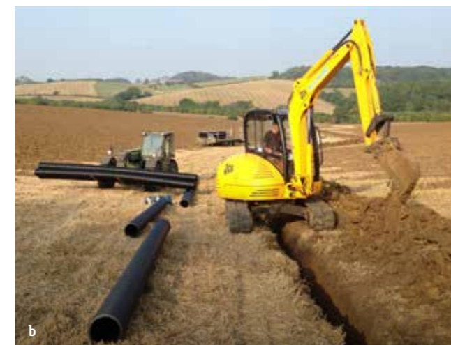
Figure 13: Some measures to control undesirable water-movements may use conventional techniques. (a) In winter 2012/13 a block of arable land in the Eye Brook developed a large overland flow causing extensive soil erosion. This was due to an under-capacity field drain. (b) The old field drain was replaced by a new larger capacity field drain which eliminated the overland flow. The drain discharges into a sediment interception basin before entering the Eye Brook.
