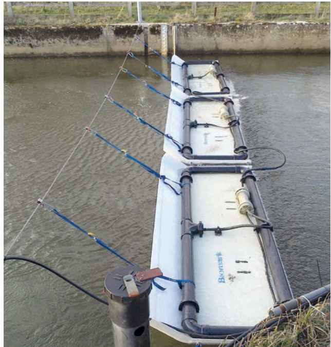
Figure 17 Floating PIT-tag antennae are part of the PIT-tag systems on the River Frome at East Stoke
