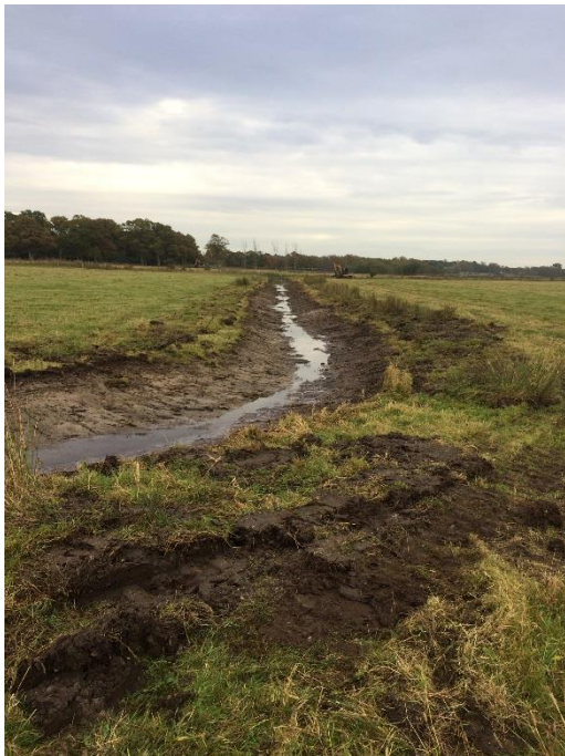
Examples of ditch creation and reprofiling at Watton's Ford.
