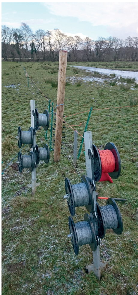
Figure 2: Main corner post with 2 x four-line reel posts holding metal wire reels and orange polywire, facing in the direction of the adjacent corner post
