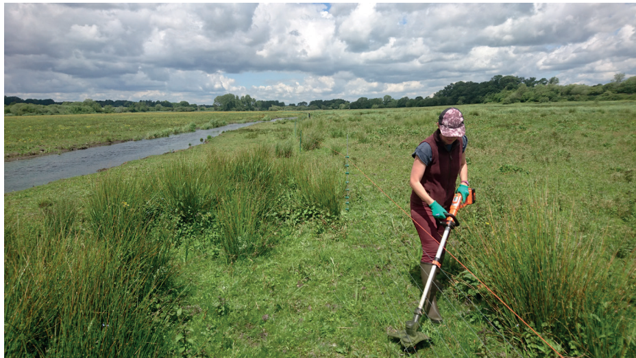
Figure 7: Strimming of vegetation under fence wires to mitigate against voltage loss
