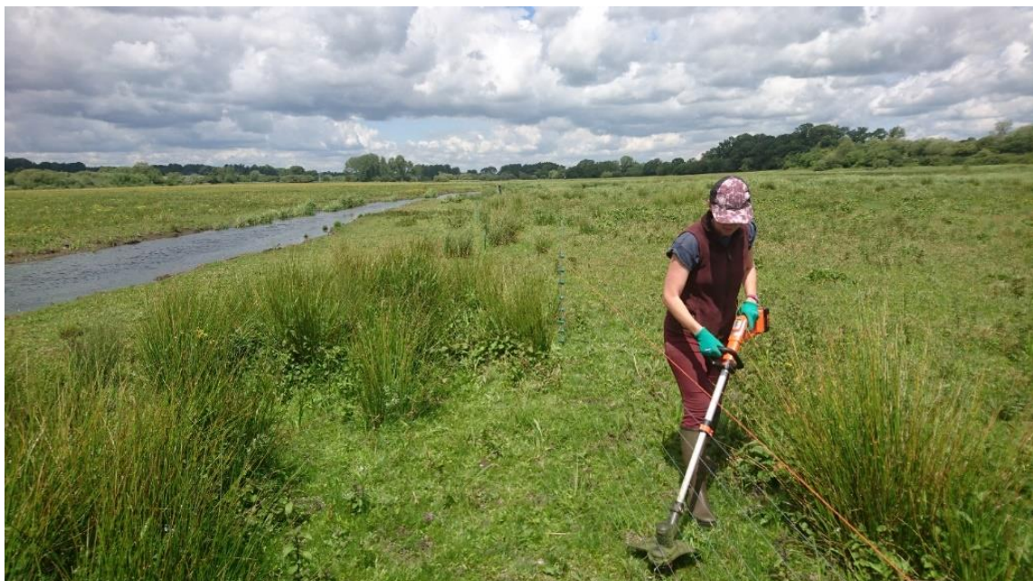
Figure 8 Strimming of vegetation under fence wires to mitigate against voltage loss
