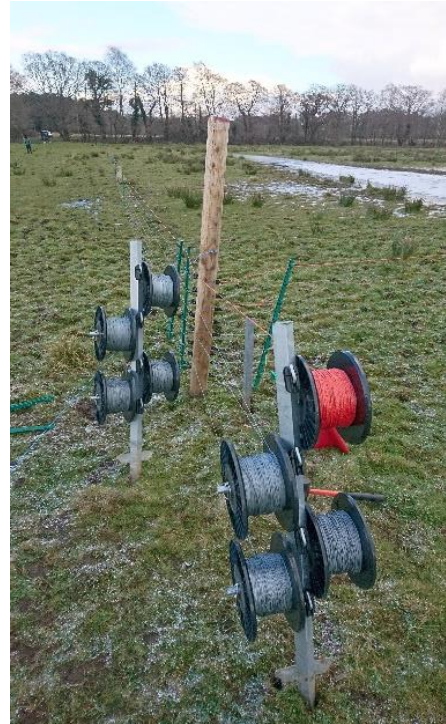
Figure 6 Main corner post with 2 x four-line reel posts holding metal wire reels.
