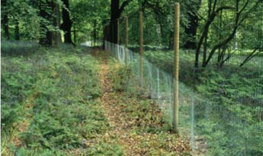
The fence should consist of two meshes. Small mesh at the bottom and bigger mesh at the top.
