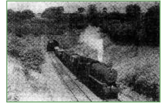
The south end of the railway tunnel at East Norton, 1958. Photo courtesy of Haywood Bishop.
