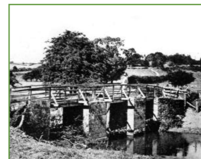
The bridge in the 1930s...
