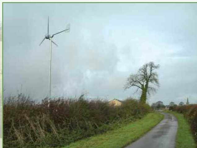
Modern wind turbine at Tilton
