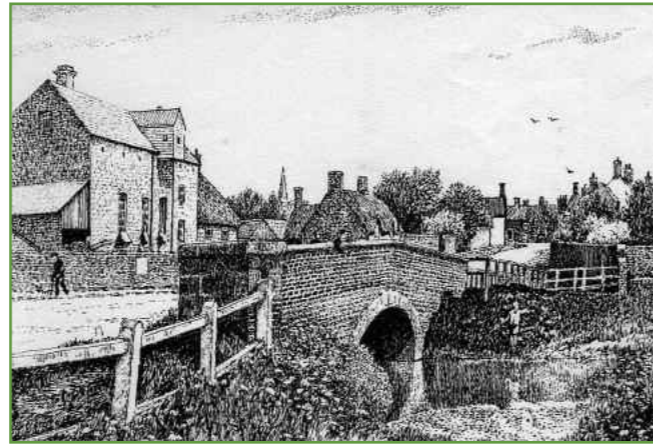
Caldecott Mill drawn by JRH Prophet from an early twentieth century photograph.
