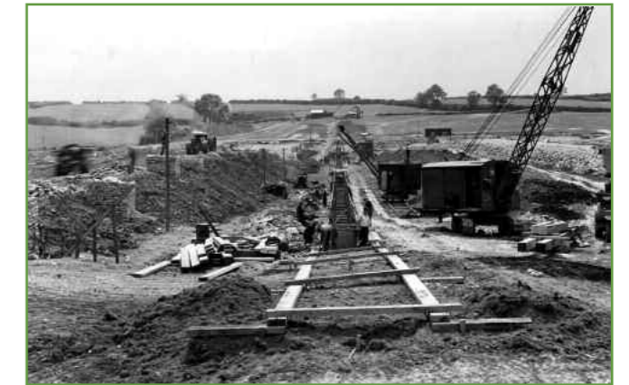
The dam under construction in the late 1930s.
