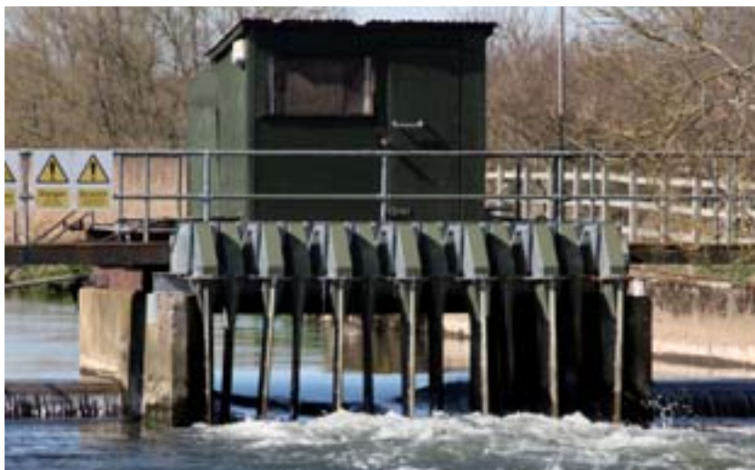
PIT tag data are collected by detection vanes mounted on the main river counter.
