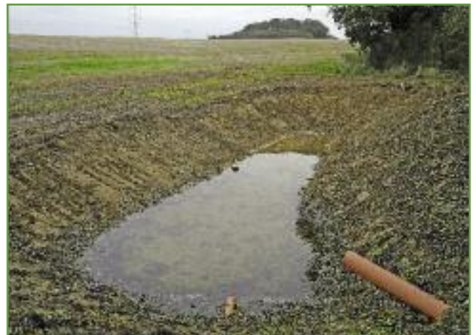
Field drain interceptor ponds have been created to trap sediment and nutrients before they enter the stream.
