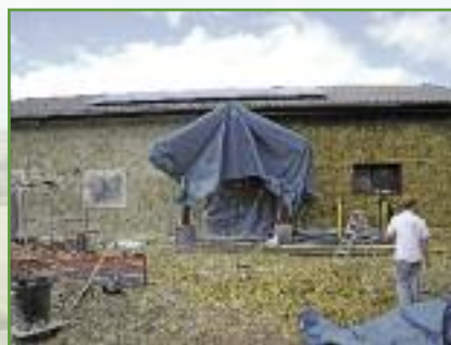
The visitor centre under construction
