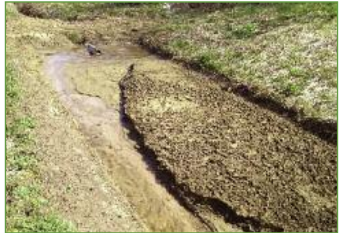
A ditch dam holds back water and traps soil washed from arable fields.
