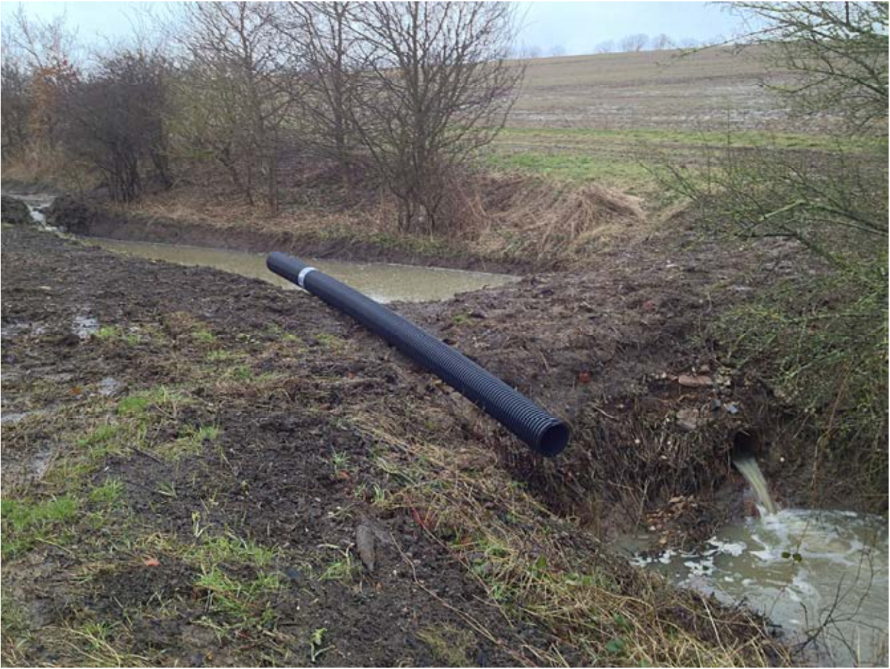
Figure 56. Large earth-bunded ditch interceptor under construction.
