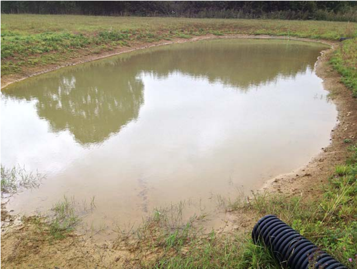
Figure 55. Detail of inlet pipe in a flood detention pond on the Eye Brook (downstream of detention pond in Figure 4). The outlet pipe is visible at the top right of the photograph.
