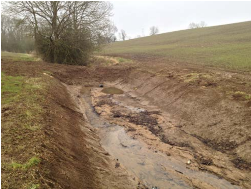
Figure 51. Large earth-bunded ditch. The picture shows the bund before being 'switched on', with bottom pipe still open. This pipe is now closed and the bund retains water and sediment during high flows.
