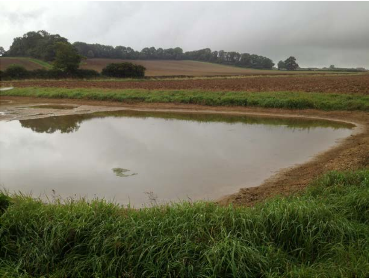
Figure 54. Flood storage basins. This flood storage basin detains water temporarily from the ditch draining the arable area behind the site, including the land upslope to the woodland. Figure 55 below shows detail of a second, adjacent, flow detention pond.
