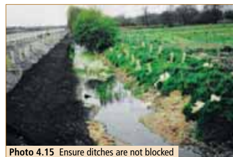
Photo 4.15 Ensure ditches are not blocked
